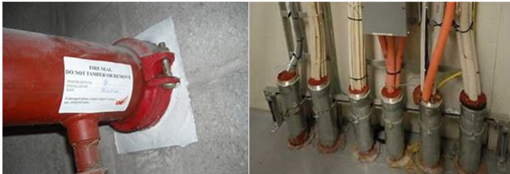
Figure 4: Fire Stopping Through Walls and Floors
